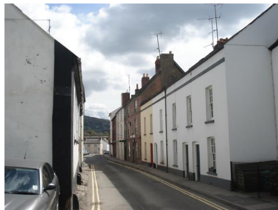
Fig.27 St John's Street, the subtle but effective variation in materials and material use greatly adds to the special character of this part of the conservation area
