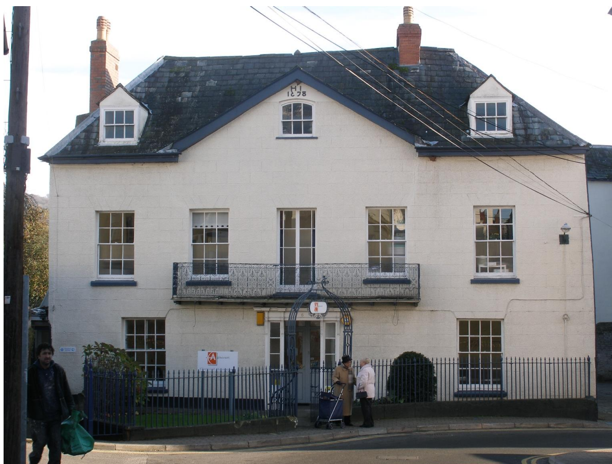
Fig.120 No 6 Agincourt Street. It is dated 1678, as can be seen in the pediment. Classical symmetry is apparent in the design, although most of the windows are later.
