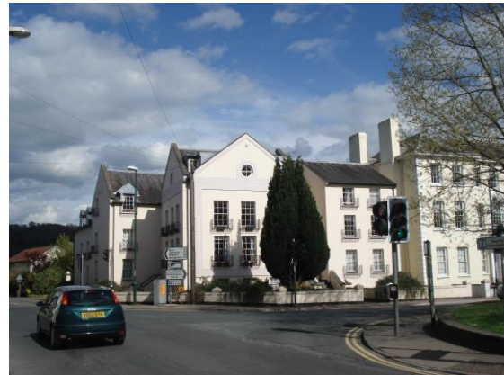
Fig.101 New buildings to the junction of Monk Street and Dixton Road maintain the important enclosure to this junction and building line to these major routes
