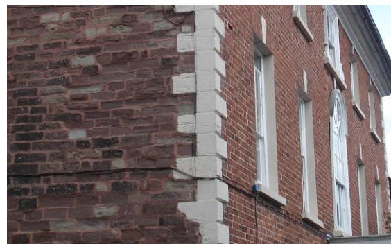
Fig.192 St James' House, a 16 th century stone building re-fronted in brick in the 18 th century.
