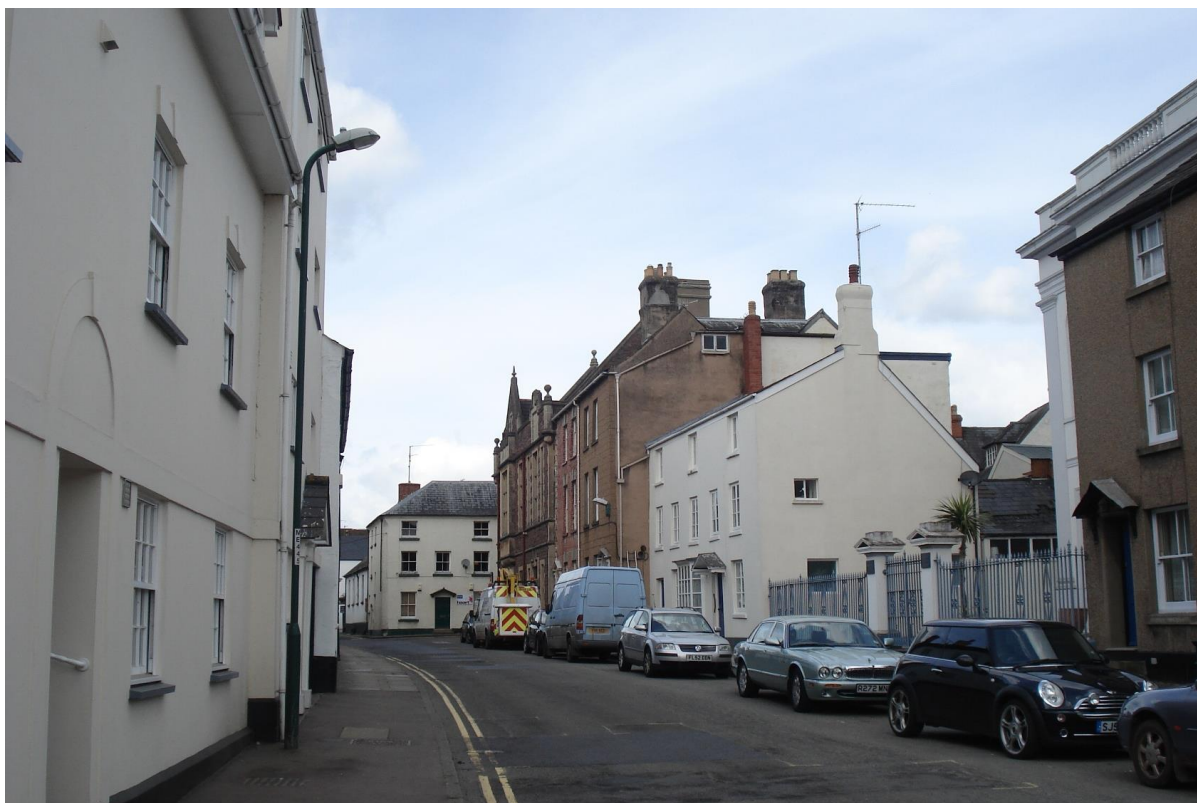
Fig.17 The street line is often continued with railings and boundary walls – seen here looking north-west along Glendower Street
