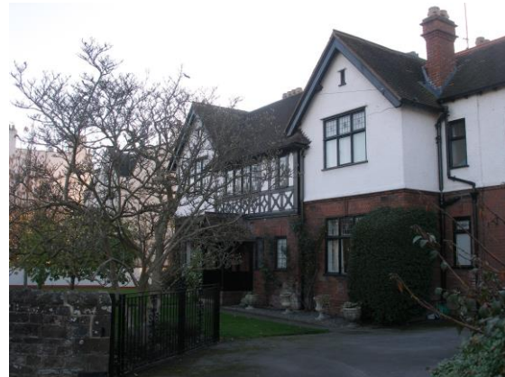
Fig.169 The Gables Hereford Road, one of a handful of spacious houses of the Domestic Revival dating from the turn of the 19 th /20 th centuries.
