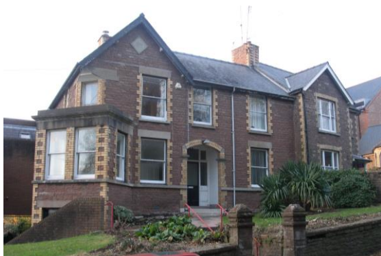
Fig.159 Further down the hill, this house, dated 1899, became part of the School. Its bay windows, are angled to take advantage of the sun and the view.
