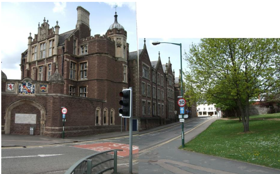
Fig.64 The exuberance and embellishment of the built form and the use of tall chimneys and well-defined gables characterises a number of the buildings forming part of the boys school complex
