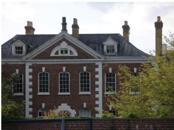
Fig.126 The earlier, mid-18 th century, rear elevation of Cornwall House, facing south east to what are now car parks.
