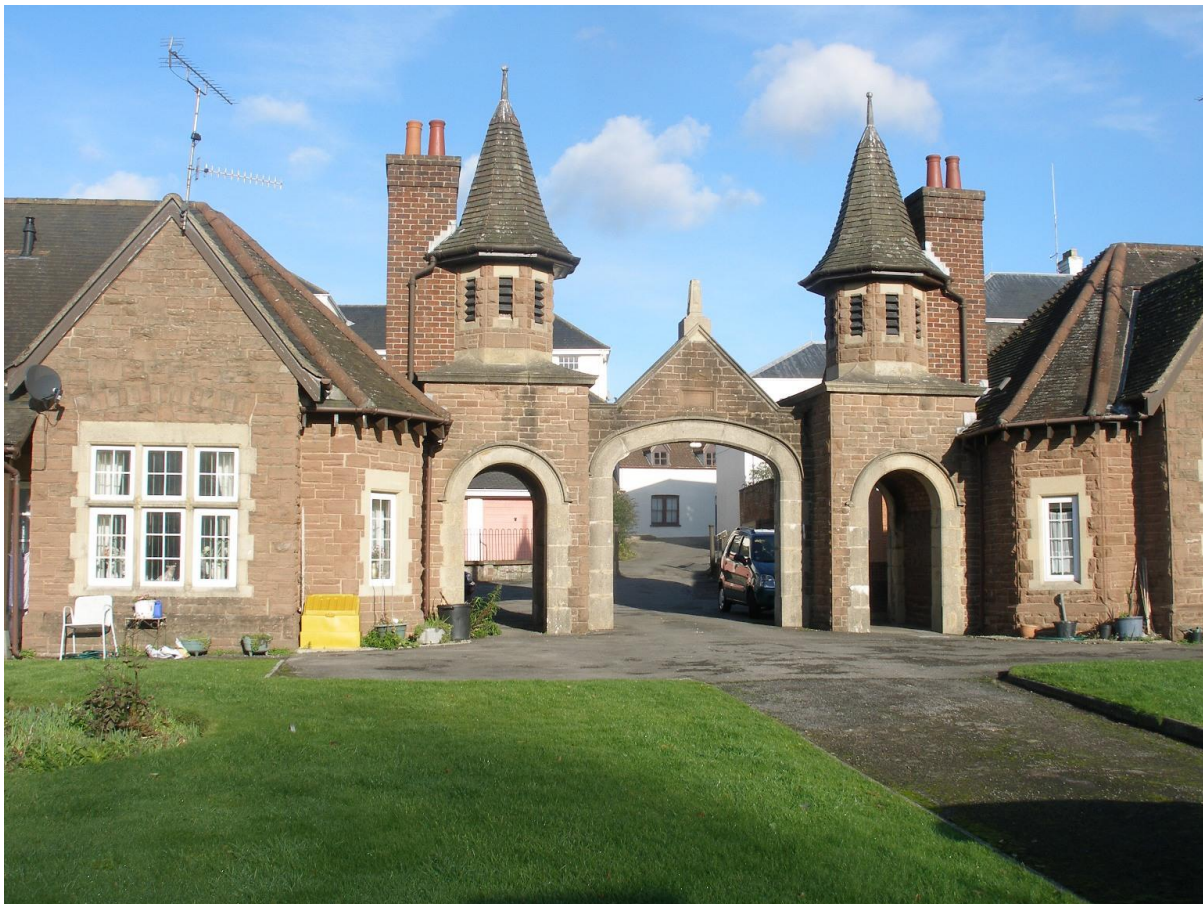
Fig.172 Henry Burton Court almshouse group, whilst built in 1928 has distinctively Victorian characteristics
