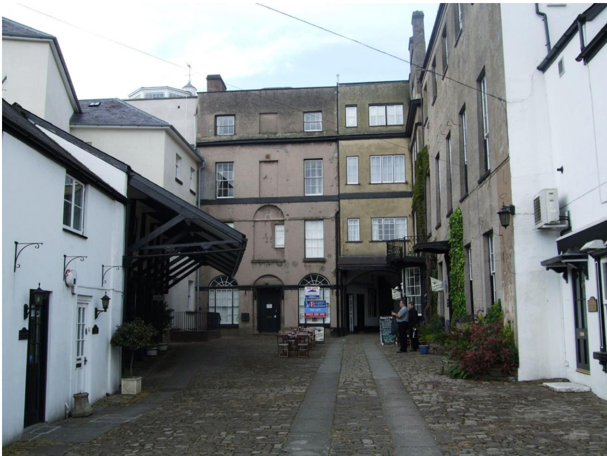
Fig.32 The courtyard to the Beaufort Arms retains its traditional stone sett surface and carriageways finished in flag stones
