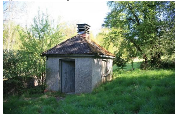
Fig.205 Mortuary building to the former cottage hospital
