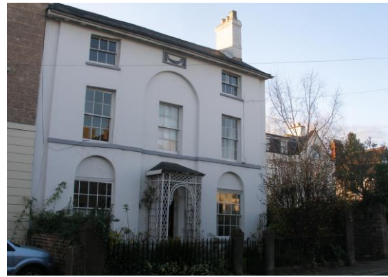
Fig.129 No. 20 Singleton House, Monk Street. A later Regency house of c 1830. The tented canopy and trelliswork of the porch offsets the formality of the overall neo-classical design.
