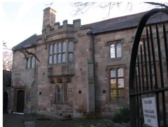
Fig.111 The remaining wing of the former Priory consists of medieval work in the lower wall and remnant sculpture. The upper parts were rebuilt in the 19 th century.
