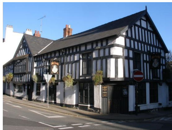
Fig.118 The Queen's Head, c1630. The gabled crosswing is the earliest visible survival of its original construction
