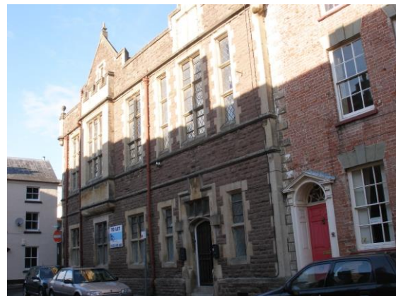
Fig.153 The Nelson Rooms, on the corner of Glendower Street and Agincourt Street continues the theme of institutional buildings designed in the Gothic Revival style and constructed in red sandstone with Bath stone dressings.
