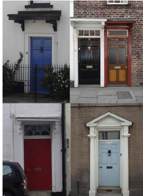
Fig.30 Examples of doorcases, brackets and hoods found in the historic core
