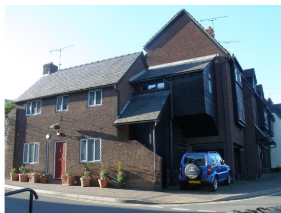
Fig.177 The Burgage, c1980s, an interesting handling of a tight corner site off Dixton Road, to create a higher density housing scheme
