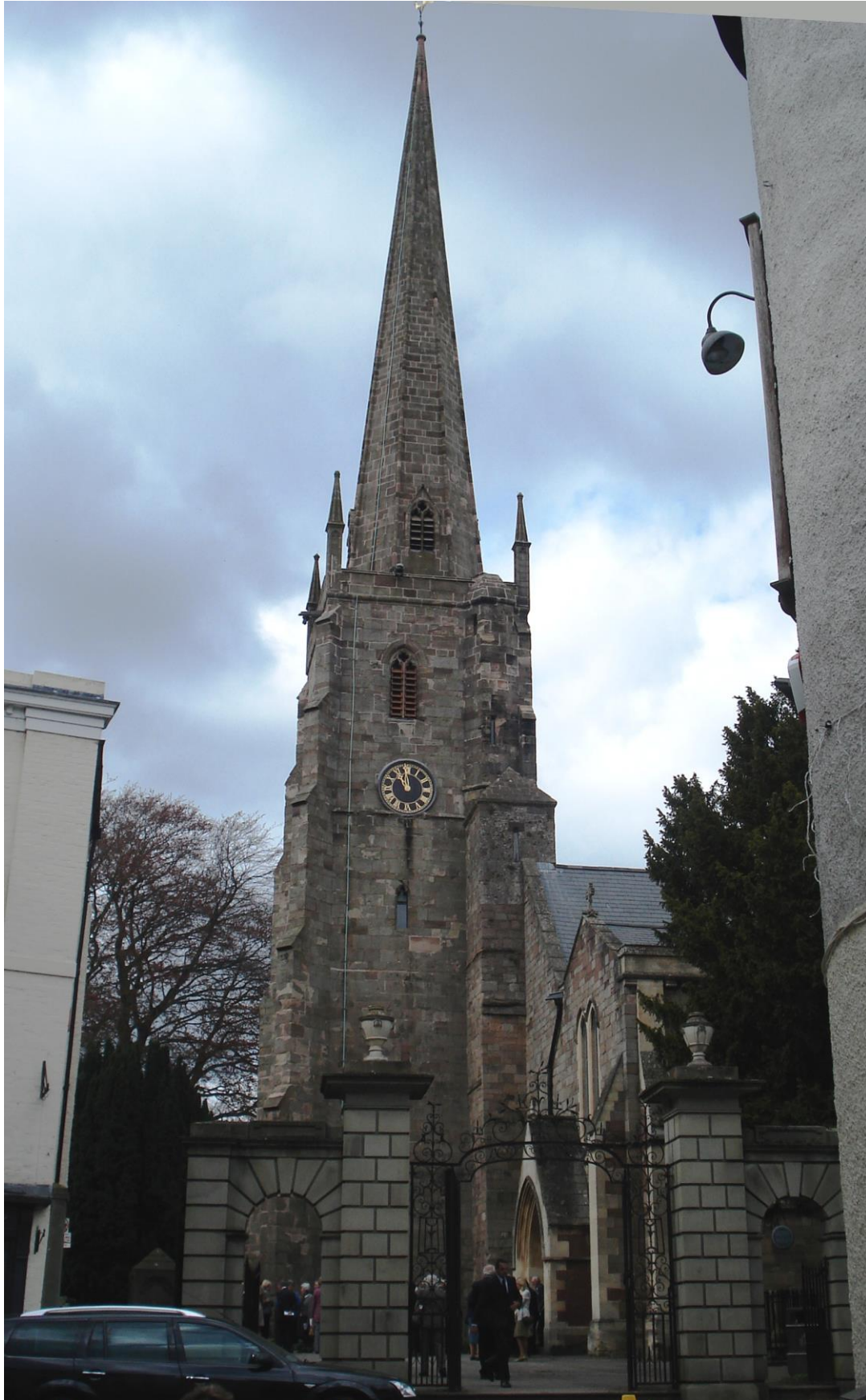
Fig.36 The gates, screen and gate piers to St Mary's church are an important local feature in the street scene
