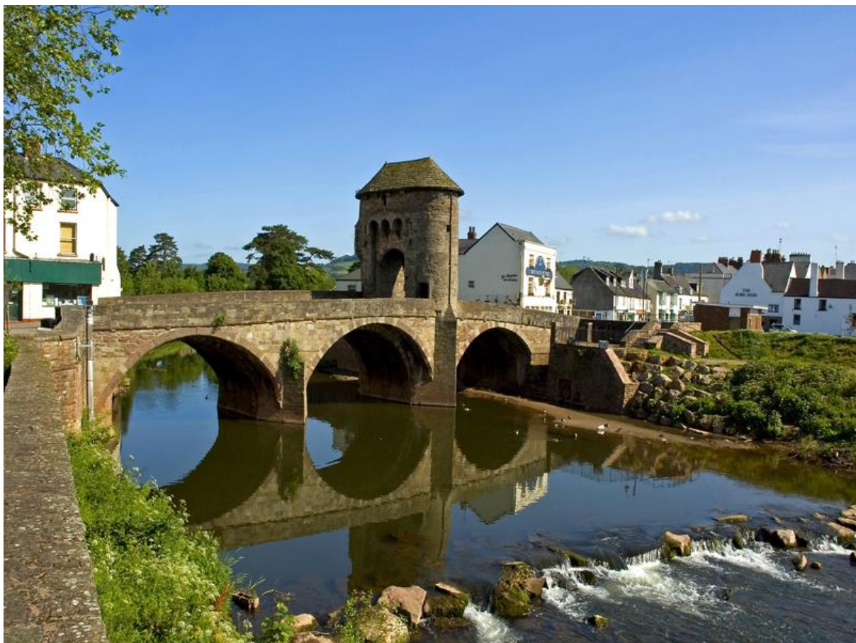
Fig.62 Monnow Bridge marking the entrance to the town from Overmonnow
