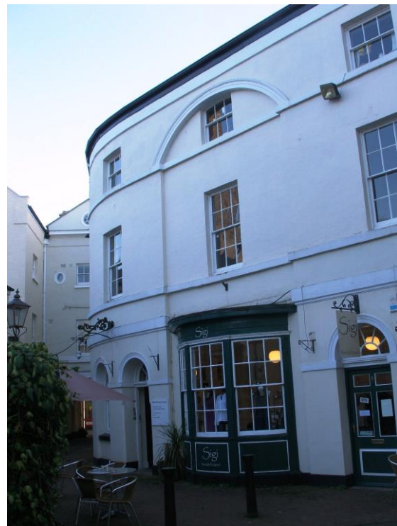
Fig.141 White Swan Shopping Court, Maddox's handsome yardscape, linking Priory Street with Church Street.
