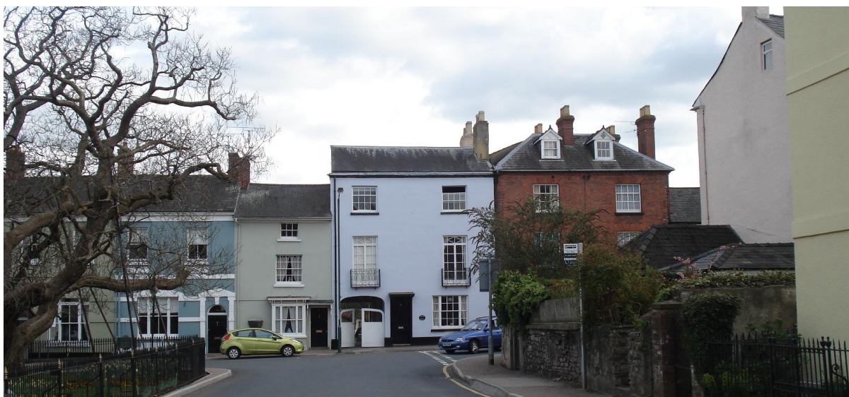
Fig.38 Architectural character around the square created by variety of well-preserved buildings of varying sizes and with painted render and brick elevations
