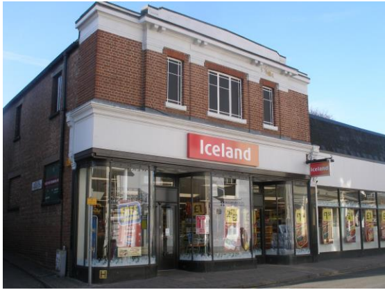
Fig.173 The former Woolworths store, designed in their inter-war corporate style. Its details, glazing (both ground and 1 st floor) and shopfront are remarkably intact, demonstrating the well considered elevational design.
