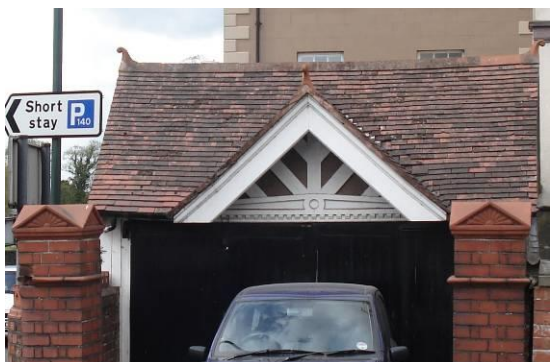
Fig.194 This Edwardian garage retains its plain clay tile roof.
