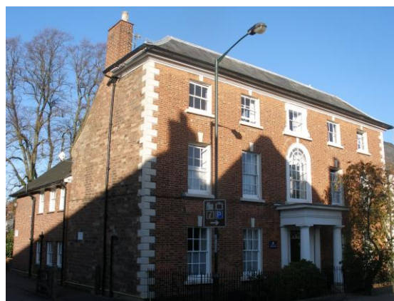
Fig.122 St James' House. Georgian refronting of a 16 th century house, as can be seen from the side.
