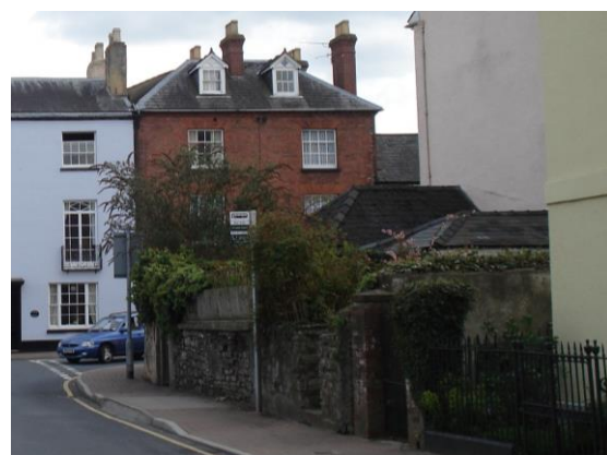
Fig.40 Boundary walls and railings maintain the line of the street where buildings are set back or gardens front streets – southern edge to St James' Square
