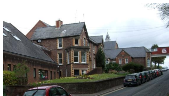
Fig.74 Buildings are generally orientated to the roadside but with features such as bays facing out to views across the town
